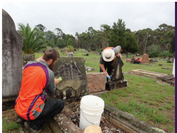
PHOTO: The RGCRT Monumental-Heritage team completing maintenance work on WW1 graves, as a part of our WW1 unofficial war graves project. Works included re-tapping lead lettering, re-attaching fallen inscription plaques, re-installing fallen monuments, removing overgrowth, and hand-cleaning inscriptions.
