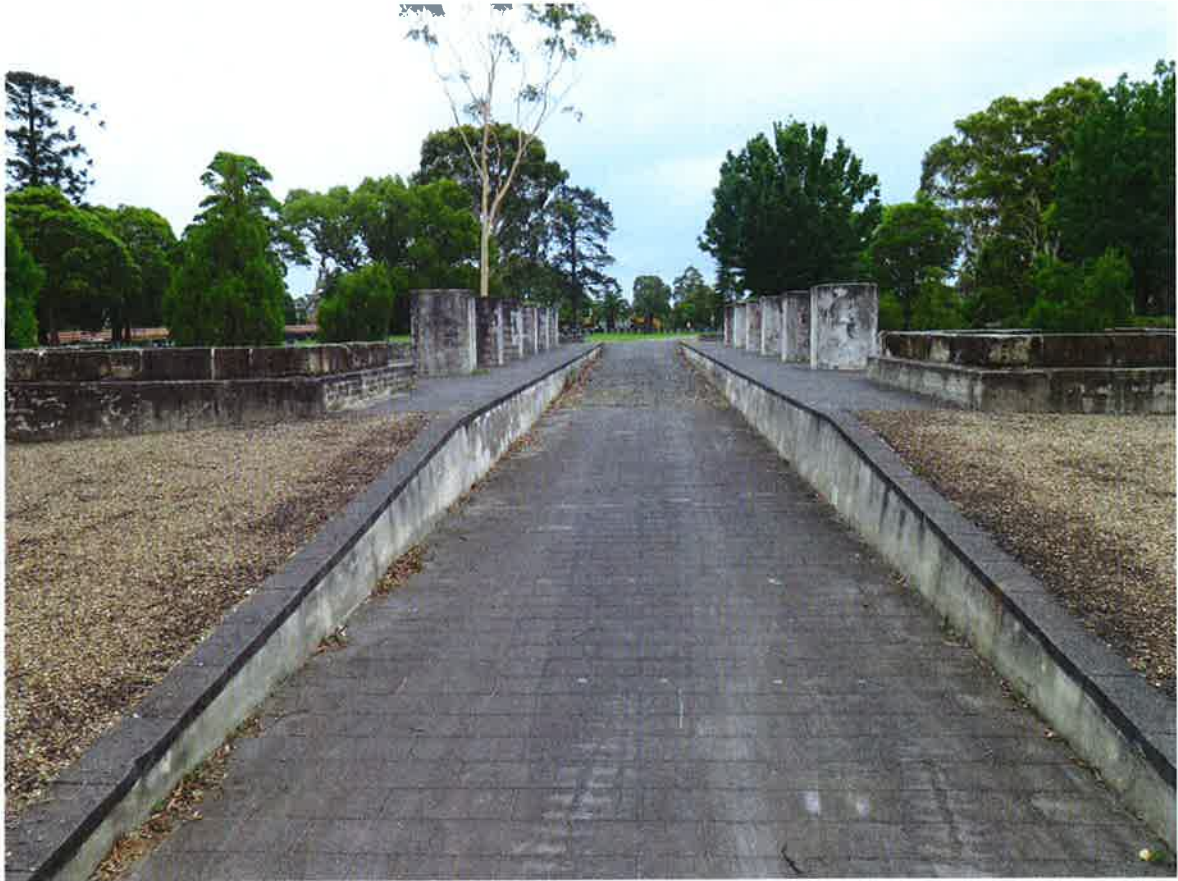
Figure 8.3 Works were undertaken to the site of Mortuary Station 1 in 1999, including exposing platform footings and the construction of concrete columns denoting the former station's original location. (Source: GML Heritage, 2015)
